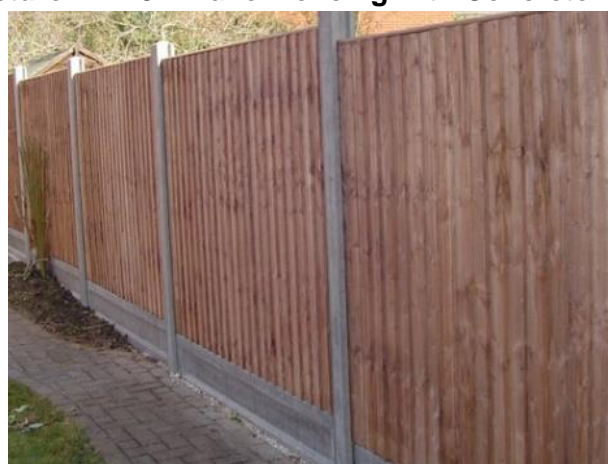
Picture 2 - 1.8m Panel Fencing with Concrete Post
